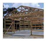
Post Frame suited to 24' to 60' spans with typical maximum height of 16'. Wider spans and large doors quickly add cost. Ideal for smaller more domestic style buildings, barn homes, and smaller commercial buildings.
